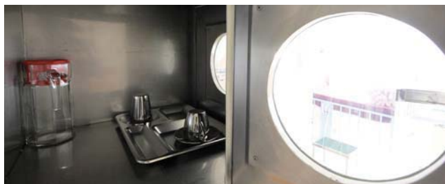
Pass Box (Safety Box) A chamber to sterilize all the equipment & materials before entering to BMT ward
